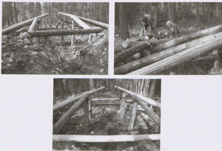
Figure 9.4 The pithouse at Vallican under construction. Note the large debarked cedar log superstructure and the trenches dug to add additional air ventilation.
